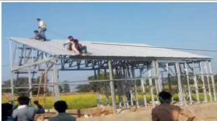
Unsafe, unsecured roof workers at a PV installation site
